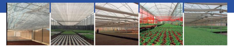
• Windows: The function of the windows is to assist in the exchange of internal air in the greenhouse, reducing the temperature and improving the quality of the air due to the exchanges! The windows can still be activated manually or motorized.
